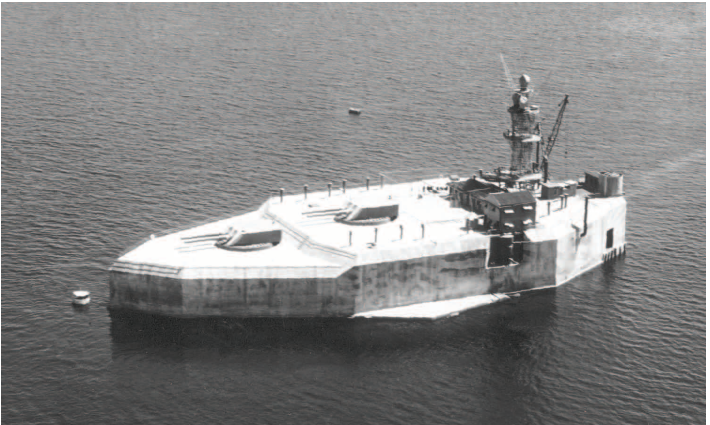
FIG. 16 Arthur Smith was Superintendent of Construction at Corregidor when work commenced on Fort Drum. It was armed with two fourteen-inch gun batteries and four 6-inch gun batteries. US National Archives photograph.
