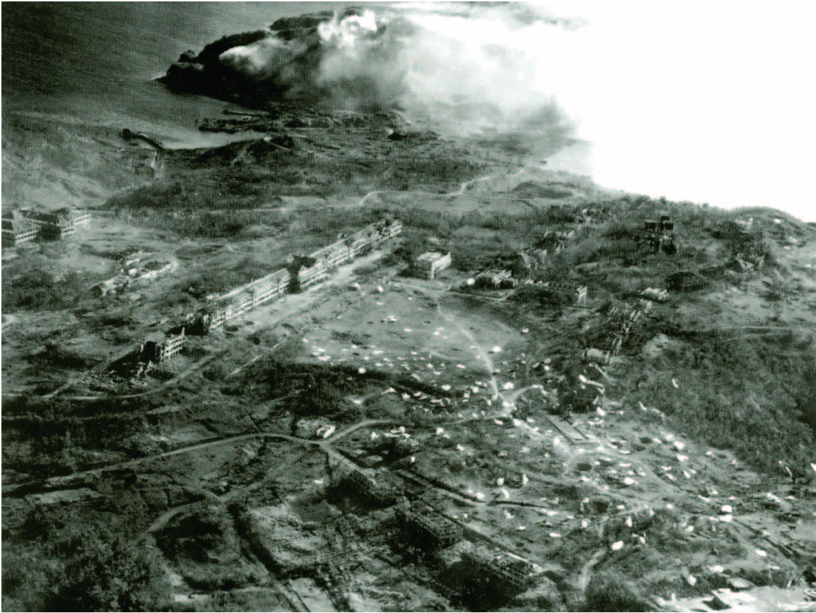
FIG. 15 Construction of the Mile-Long Barracks started in 1909 when Arthur L. Smith was Superintendent of Construction on Corregidor. The white specks in this February, 1945 photo are parachutes used by men of the US Army's 503rd Parachute Infantry Regiment who dropped in to take the island back from the Japanese. For this heroic action, they received the Presidential Unit Citation and subsequently nick-named "the Rock Regiment".
